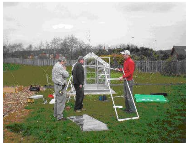
Building a greenhouse by numbers
